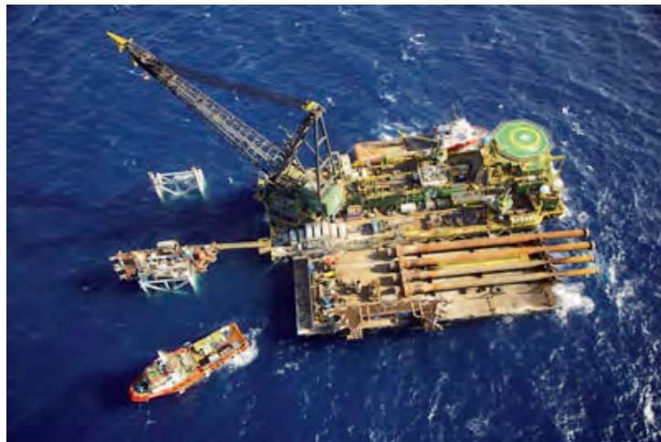
The DB30 will install the platform.
