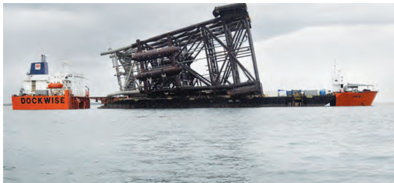
Marlin B Jacket float off in Westernport Bay.
