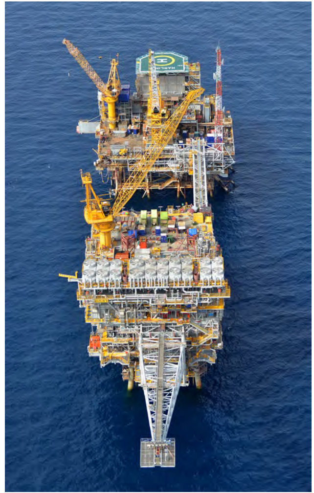
Figure 7 – Marlin B platform with all modules, flare boom and bridge installed. (Marlin A platform in background.)
