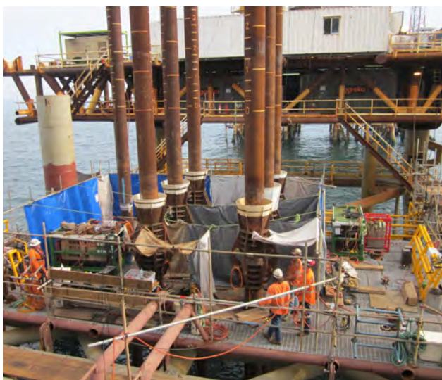
Figure 1 – Installation of Marlin B conductors.
