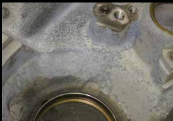
IDG housings show signs of corrosion.
