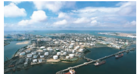
ExxonMobil's Jurong, Singapore, base stock refinery (above) has been serving the Asia-Pacific market with additional Group II capacity since the refinery's expansion was completed in early 2015.
