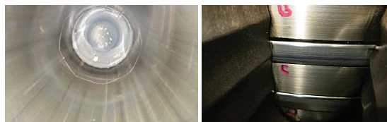
Unit 1 at interim inspection
